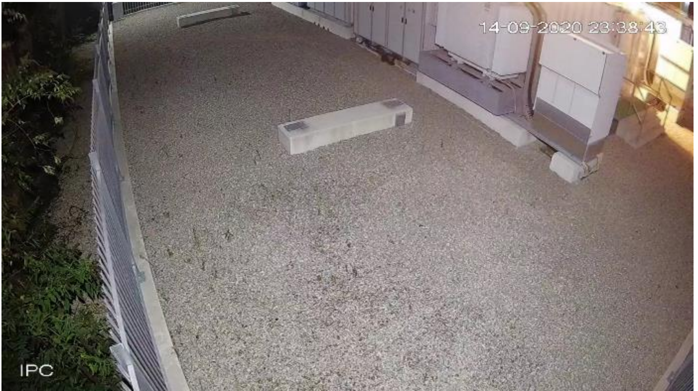
External CCTV at point of blast for the door fails
