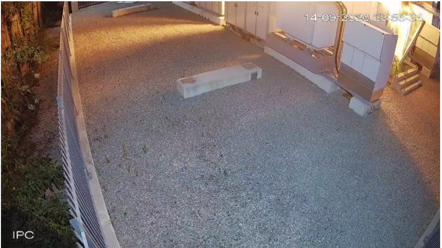
External CCTV showing the door being blown open and the smaller door coming detached
