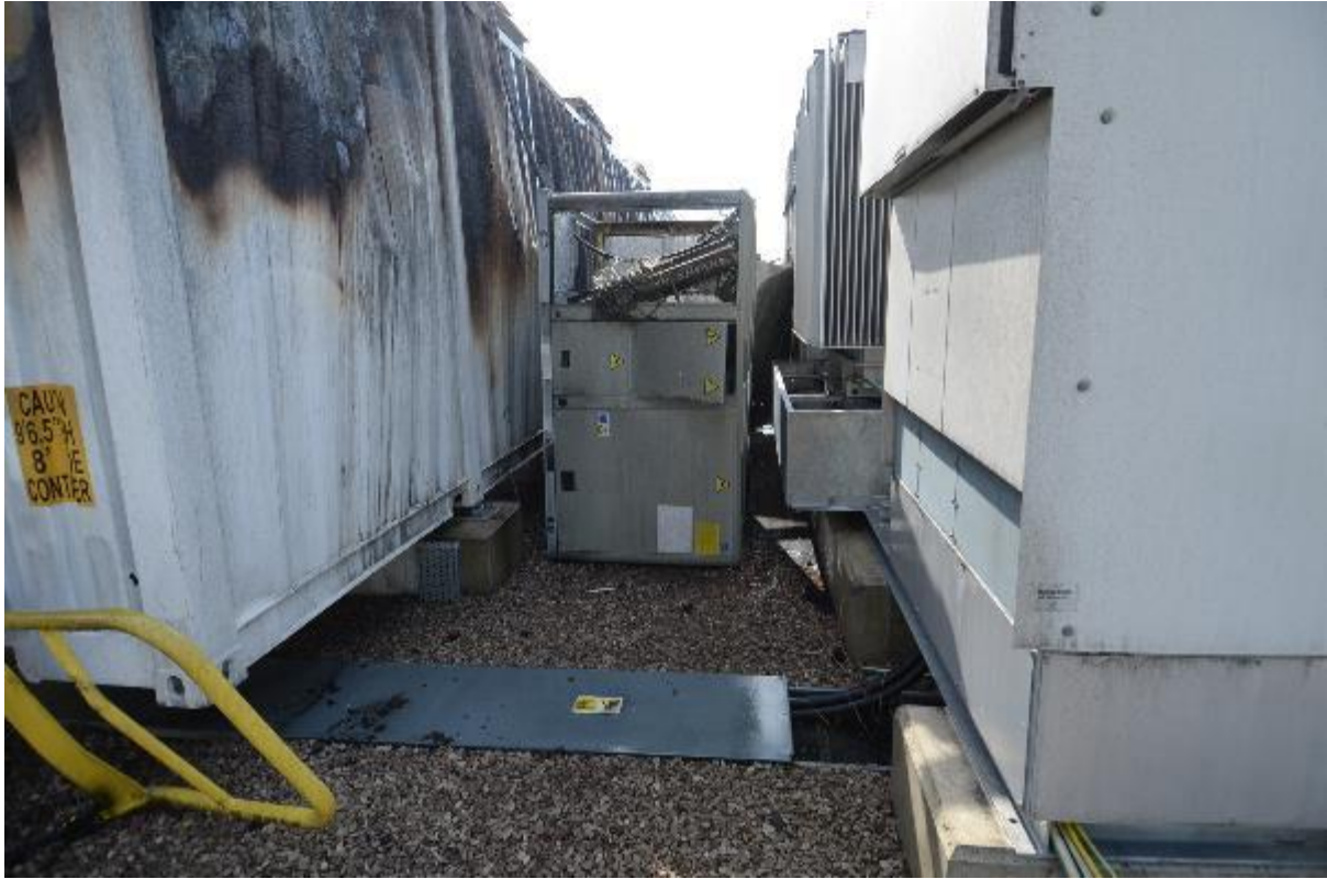
Right aspect of container one
