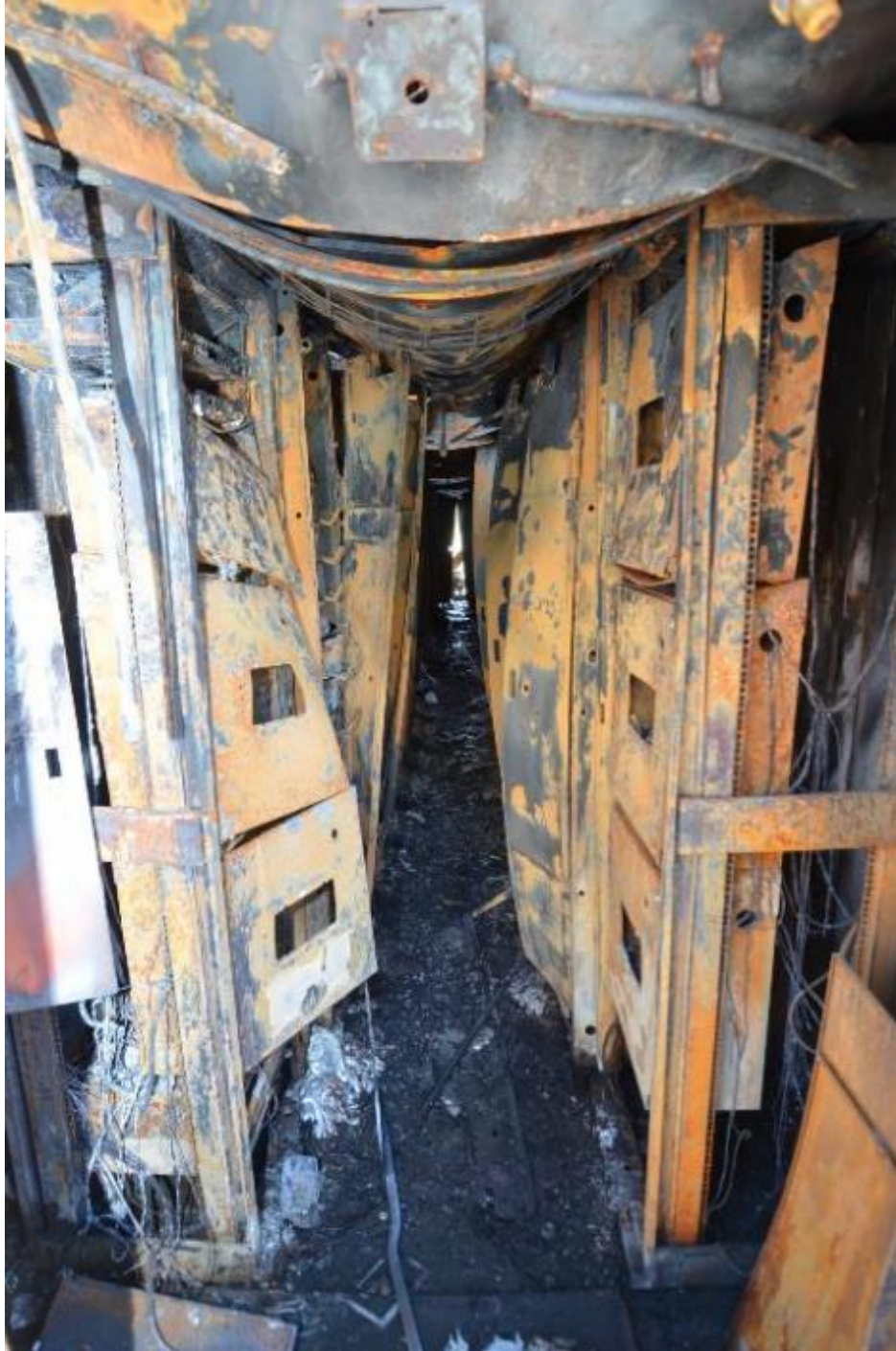
Internal view of container one from the Fisheries side
